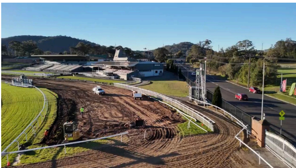
Gosford Track Progress.
